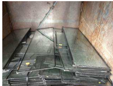
Stacking the window in skip.
