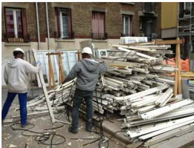
Dismantling of windows.
