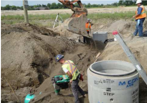
Backfilling
